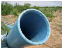
Temporary casing 3m (3 pieces)
